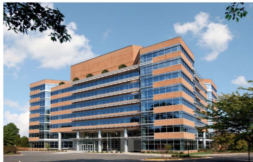
OVERALL VIEW OF NEW FACADE Overall view of new facade with light blue tinted glazing, continuous ribbon glass, and new vestibule and aluminum column wraps at entry
