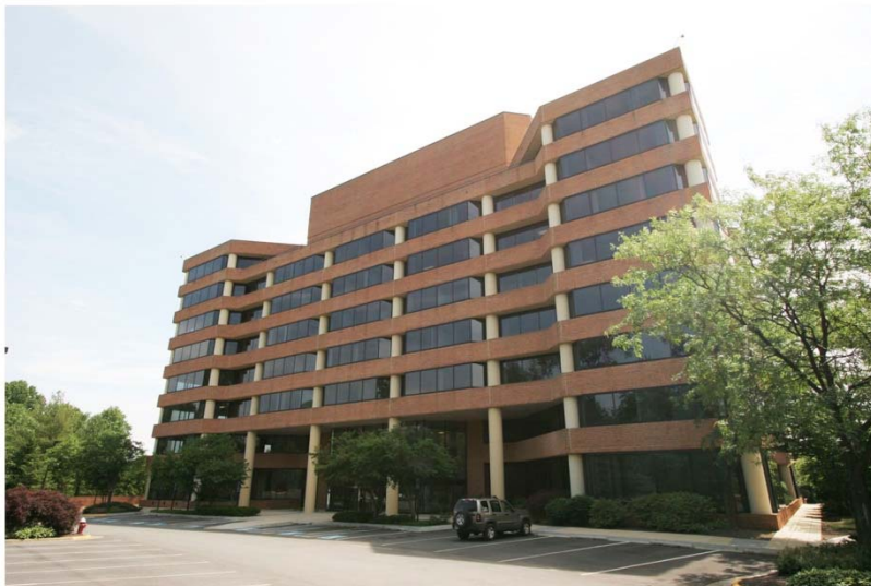
BEFORE OVERALL View of existing exterior with dark grey glass and recesses at exposed white concrete columns.
